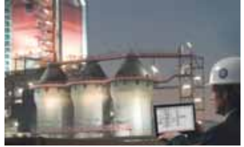
The new blast furnace 8 in Duisburg: Fitted with state-of-the-art pollution control equipment.
