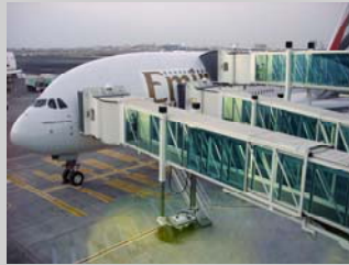
New, height-adjustable apron drive bridge for the Airbus A380
