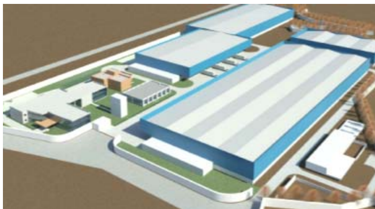
Multi-purpose facility under construction
