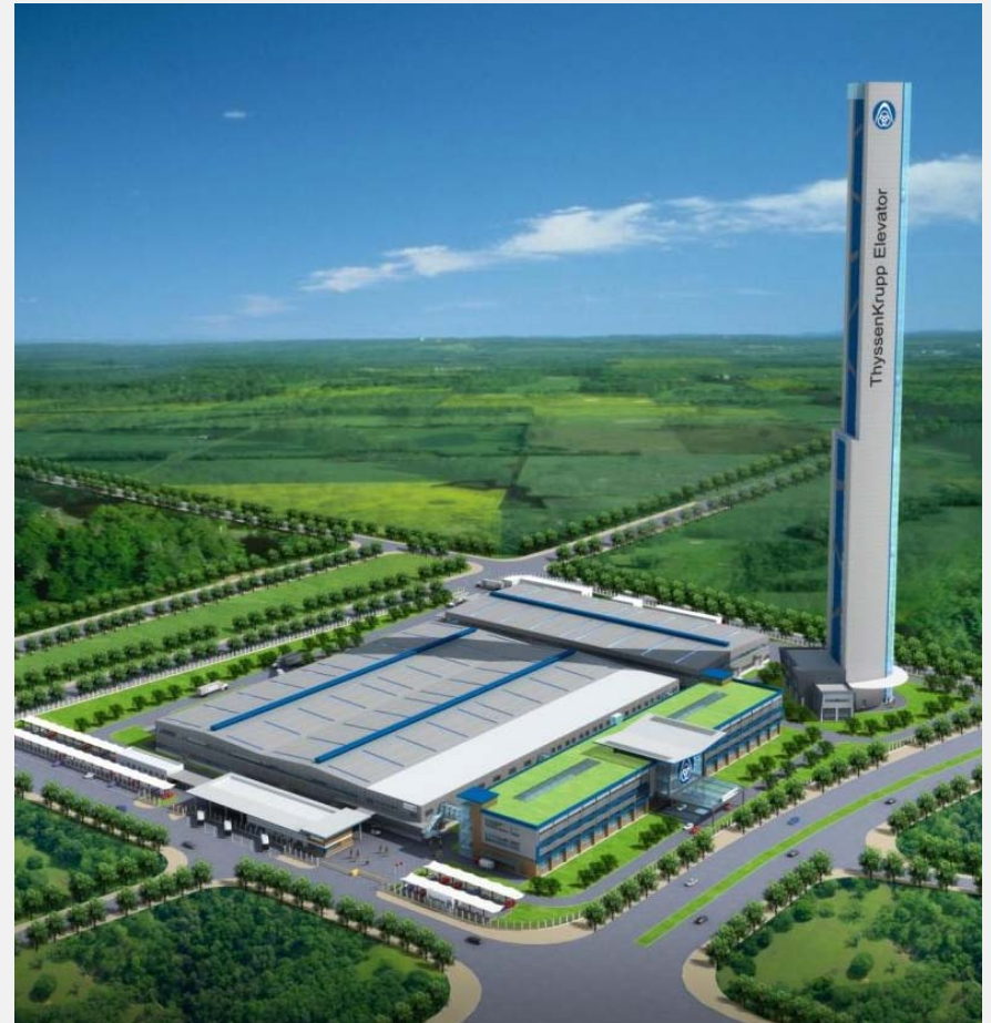
New Test Tower for Zhongshan factory
