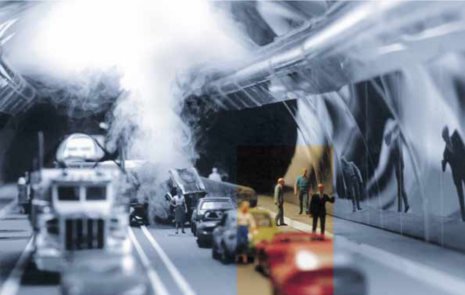
People and buildings are protected by removing smoke and heat directly from the source of the fire (Fig. 1)
